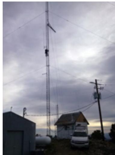
there was a program with noise on the remote base. Don, George Gallis AL7BX and Bill Stenger K6QOG went up the mountain to replace the coax and adjust inputs and output of the radio and controller. The picture is of the tower and the building on the right side of the tower houses the remote base. Bill is on the middle of the tower
