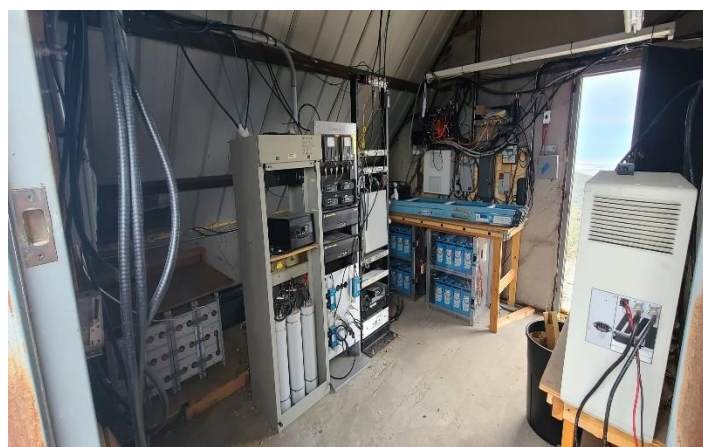
Black Mountain Repeater Site Vault Picture take by Paul Wolden (K7WEP)
