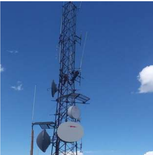
John Rice (NR7T) on right and Bruno (KG7VVN) on left making repairs. Photo by George (AL7BX)
