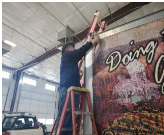
Brad (WA7HHE) prepping seams for caulking.
