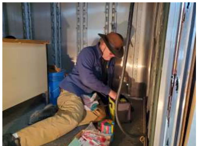
Fred (KI7TPD) prepping base of wall for insulation
