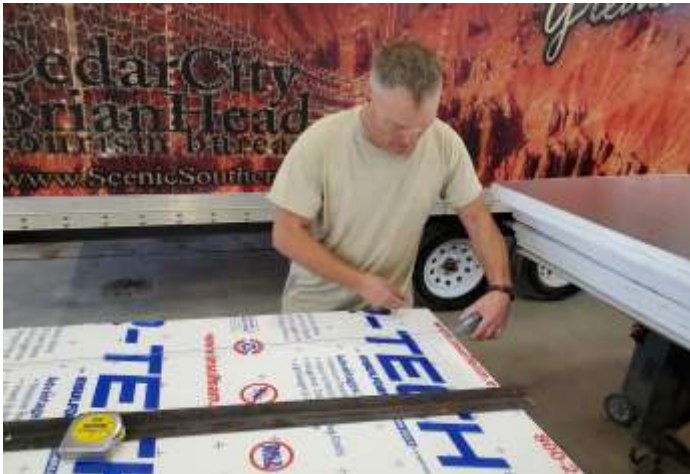
Bruno (KG7VVN) measuring insulation strips for radio room.
