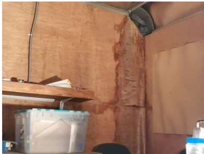
Radio room water damage
