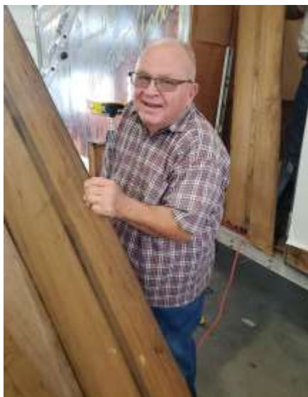
Dennis (W6DLW) stacking the removed paneling
