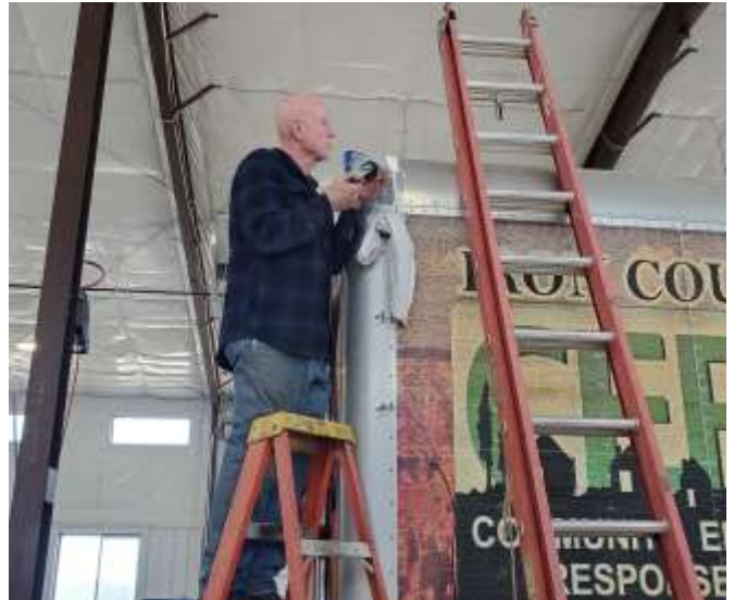
Brad caulking prepped seams at trailer front.
