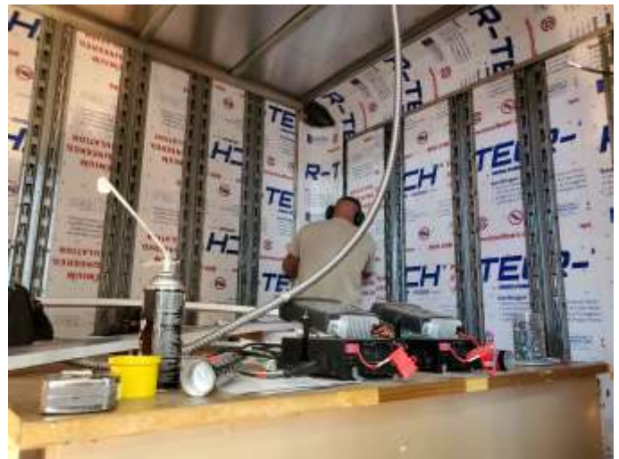
Bruno (KG7VVN) finishing the insulation install.
