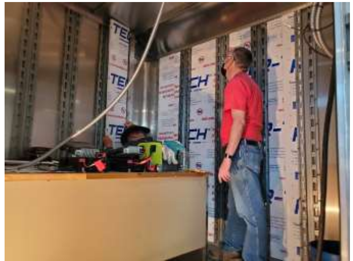
Lance waiting for the next panel of insulation for install
