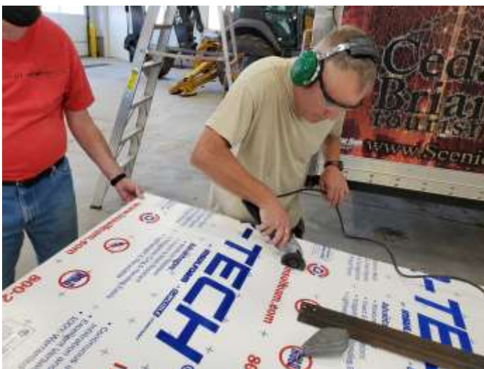
Bruno (KG7VVN) cutting the insulation for install
