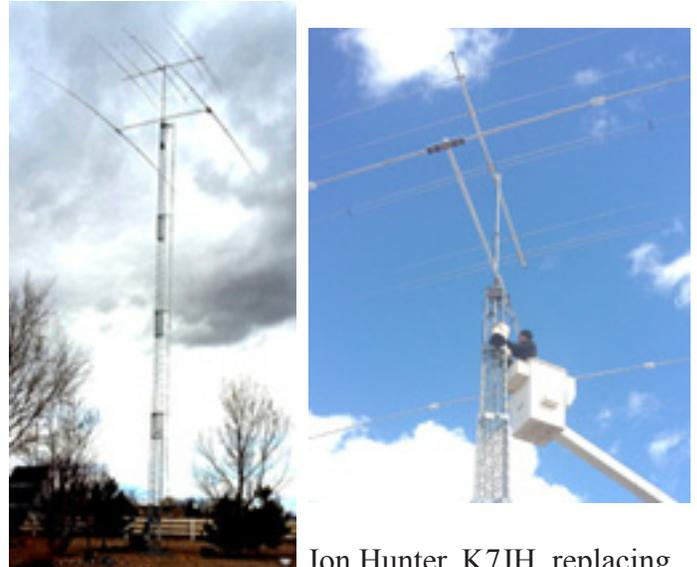
Jon Hunter, K7JH, replacing the rotor on his 40 meter two element beam. The antenna is on a 75 ft telescoping tower but still needed a bucket truck to reach the antenna.
