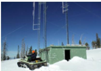
repeater site. Snow cat was the only way to get into the repeater. They added a second power supply to the rack of link transmitters and turned all links back on. Seems to be working.
