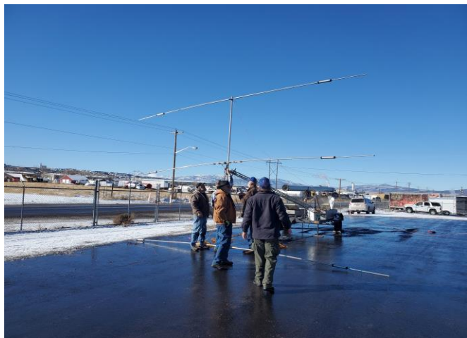
Attaching the antenna to the tower.
