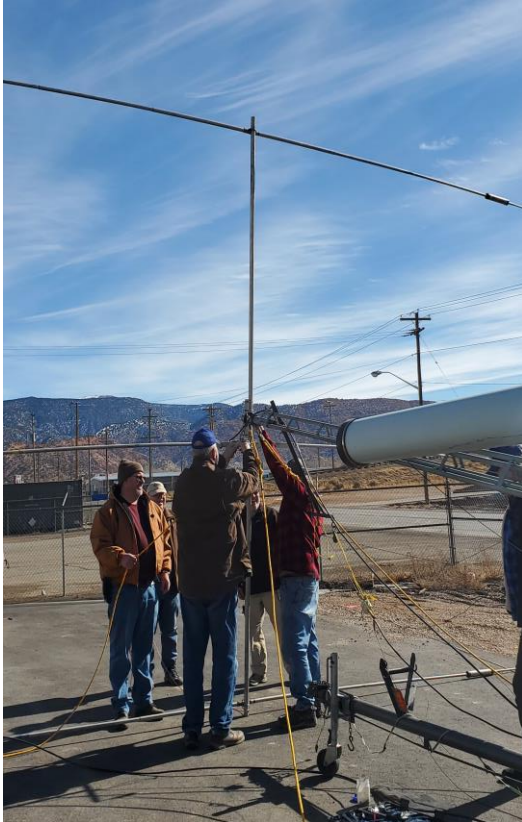
Removing the antenna.
