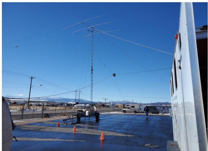
Tower & antenna up and ready for use.
