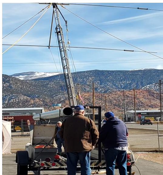
Dennis (W6DLW) lowering tower
