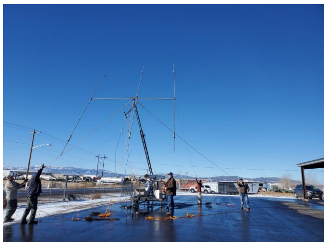
Antenna being raised to vertical position.
