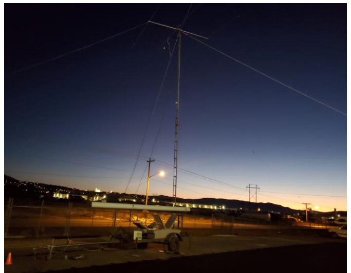
View of tower & antenna after dark.
