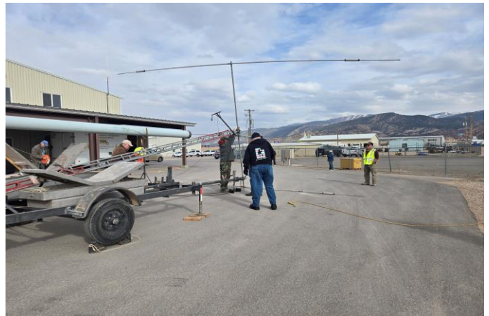
Tower is down and beam being removed from the mast.
