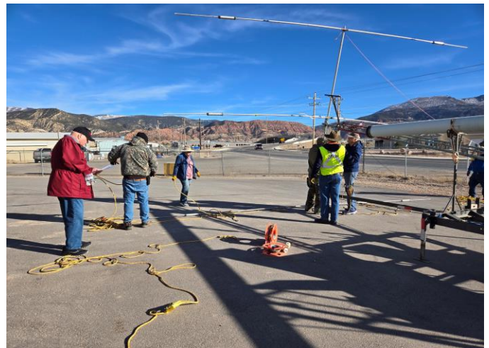
Antenna being attached to mast.
