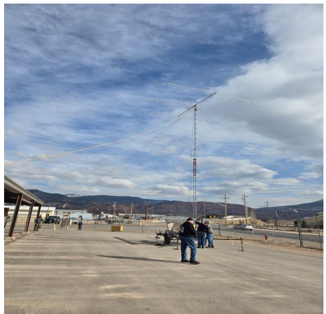
The tower is up and finishing measures are being taken.
