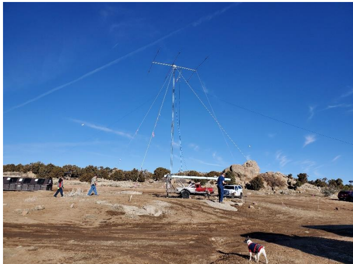
The tower is up and operational.
