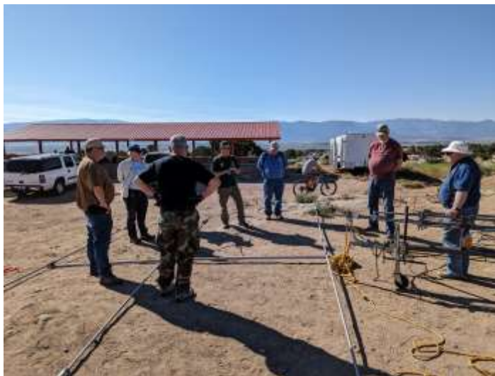
Antenna ready to be mounted to tower. Bruno (KG7VVN) providing a safety briefing.
