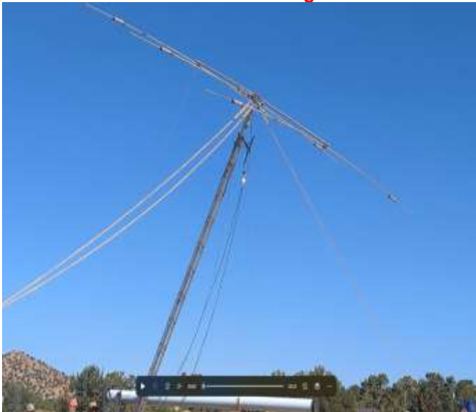
The mast is on its way up to first position before extension upward.
