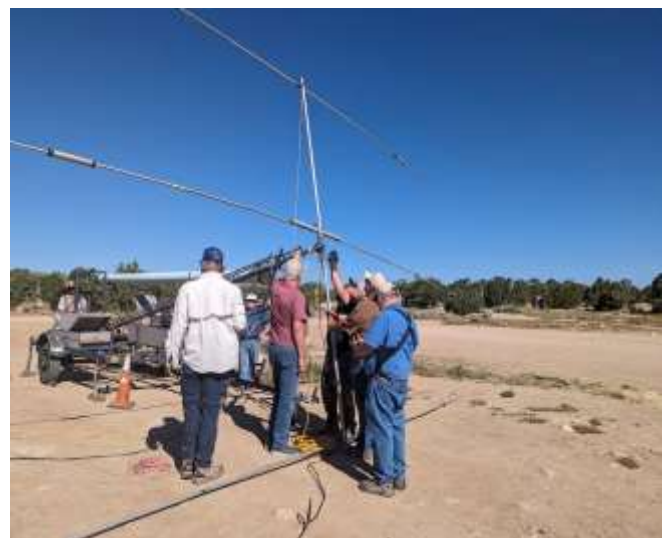
Antenna being attached to antenna mast post.
