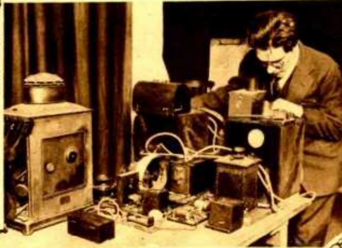
Upper Right Photo Shows Captain A. J. Hillary, Master of the Mail Boat "President," Receiving Information By Radio as to the Number of Bags of Mail on Board an Incoming Liner. Above: A Picture of a One-Kilowatt Ship Type of Quenched Spark Transmitter. This is the Most Efficient Form of Spark Transmitter, But, Due to the Greater Efficiency of C.W., They Are Being Converted Into the Latter. Aside From the Quenched Spark Gap, All the Other Apparatus is Made Use of in the Conversion.
