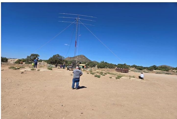
Antenna Tower and antenna now ready or use.
