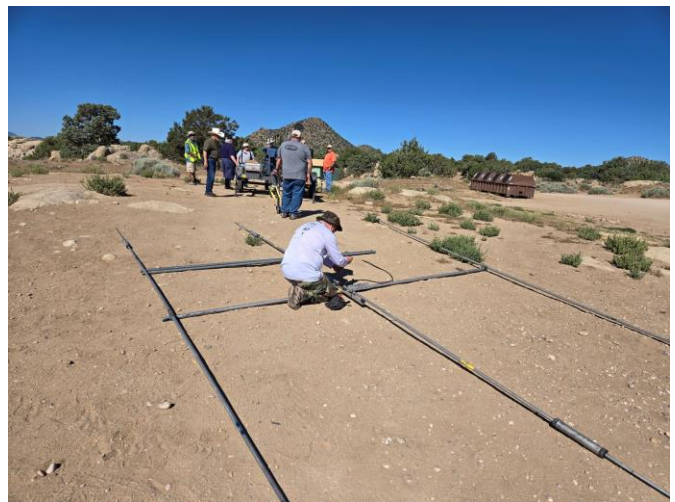
Kevin (K2MFK) assembling the beam antenna for attachment to the tower. While the guys in the background prep the trailer for stabilization.
