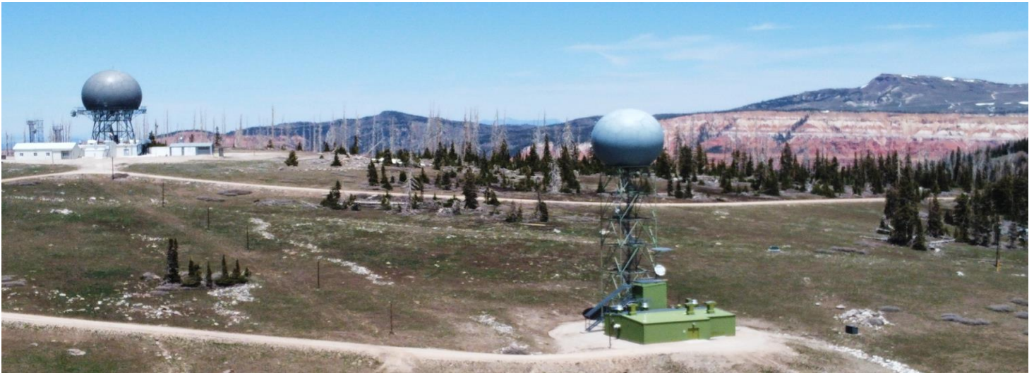
Larger dome on left is the FAA Facility structure and dome on right is the Doppler Weather Radar structure. Photo by Keith Morris.
