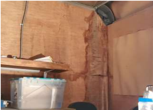
Radio room water damage.
