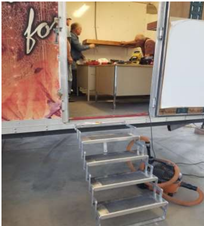
Ken (KR7KR) and Jack (KG7VEJ) reinstalling the light & Shelving Units. Note new steps in foreground.
