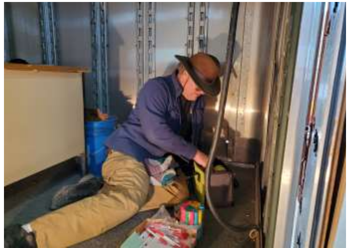
Fred (KI7TPD) prepping base of wall for insulation.
