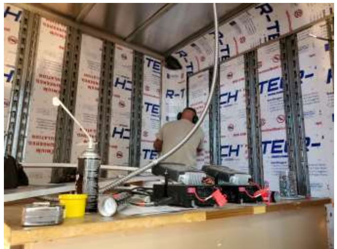
Bruno (KG7VVN) finishing the insulation install on walls.
