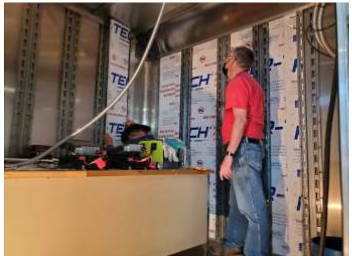
Lance (KA7J) waiting for the next panel of insulation for install.
