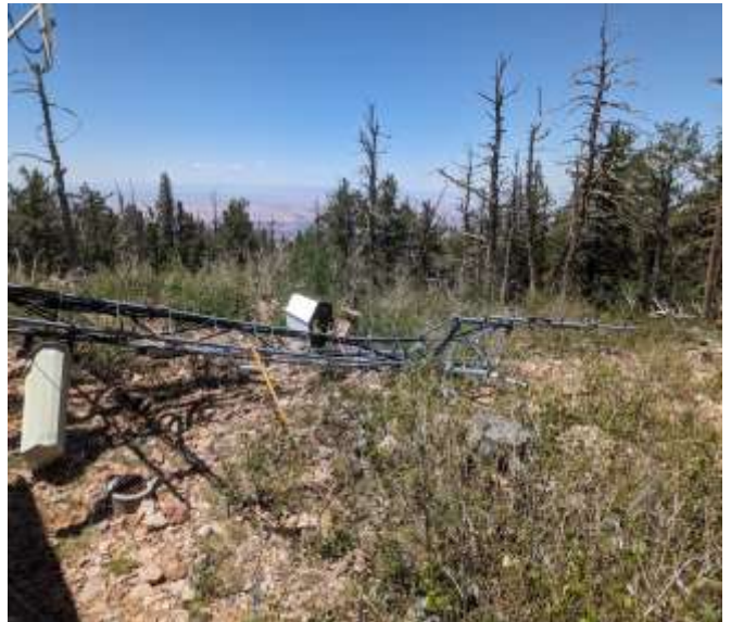
Top of Tower on ground
