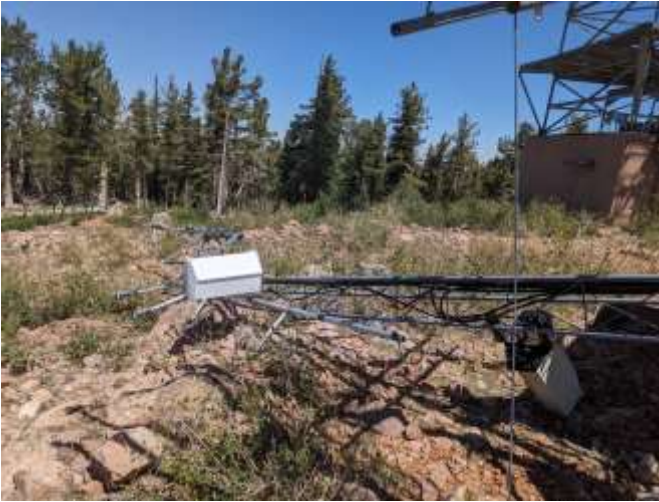
A view of top section of downed tower.
